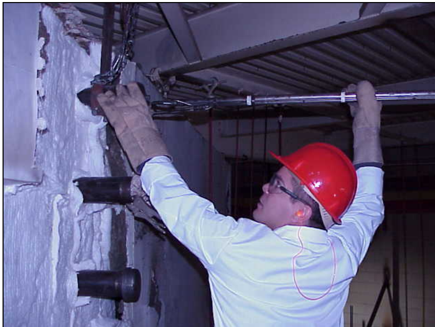
Fig. 12. Inserting particulate testing probe into breaching.
